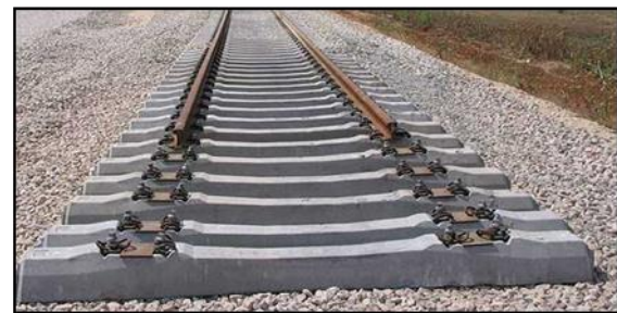
(b) Concrete Sleepers.
