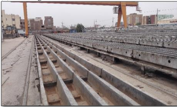
Figure 4. Preparing the frames of the strands.
